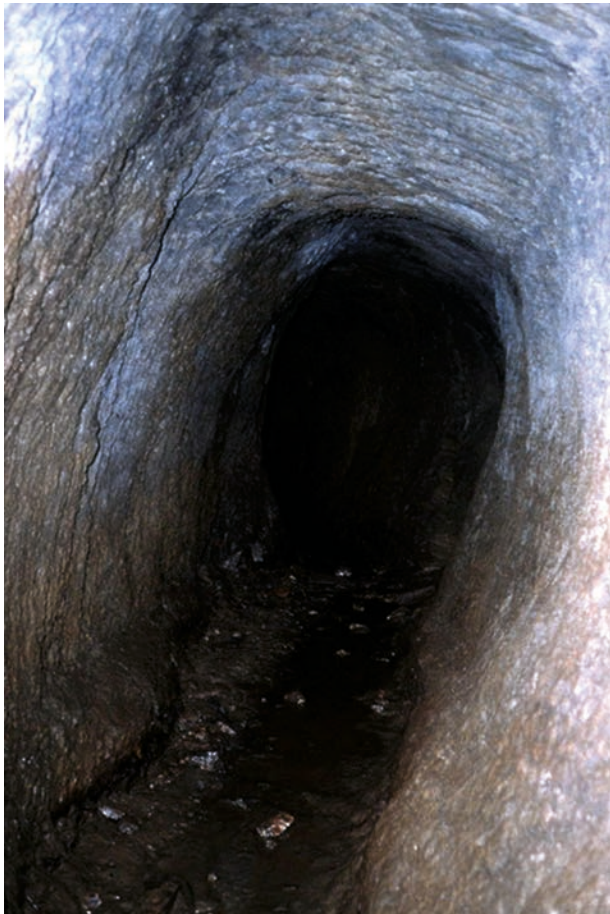
Fig. 9. View into the Venetian adit at section No. 8 in figure 8 (photo: M. Straßburger).
