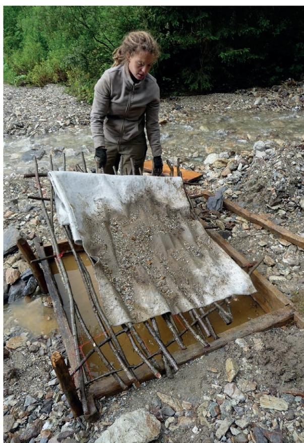
Fig. 9: Using the water-filled box with a woven wattle frame and sacking for the washing of the crushed ore in August 2016 (photo: S. Timberlake).
