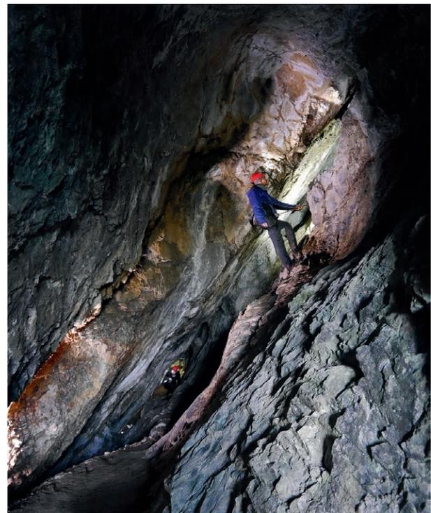
Fig. 7: A mainly fire-set mine (Gratspitz 3) at the north wall of the Gratspitz (photo: M. Scherer-Windisch).
