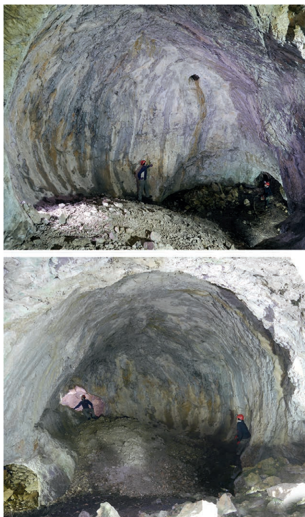
Fig. 16: The southern prehistoric fire-set part of the mine Schönbiegler Bau with chimney (photos: M. Staudt).
