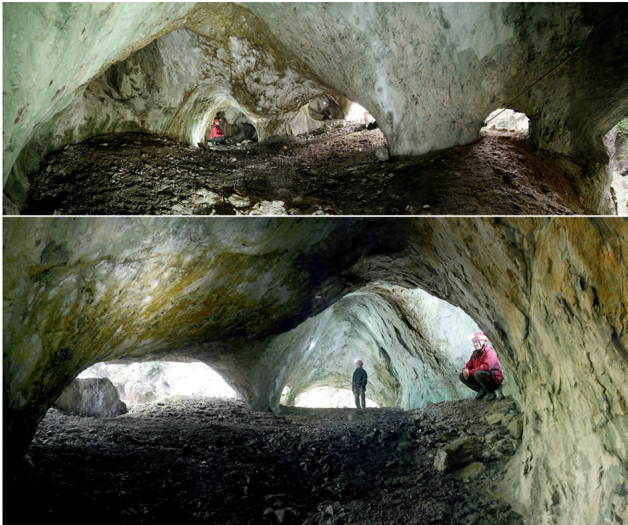
Fig. 11: Bauernzeche "upper mine", with some leftover pillars for static purposes (photos: M. Staudt).
