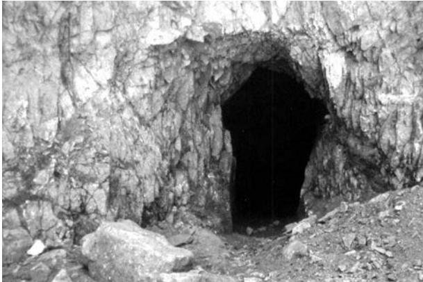
Abb. 32: Derealan-Bakır Çay: Mundloch (Photo: Bilgi 2004, 16).
