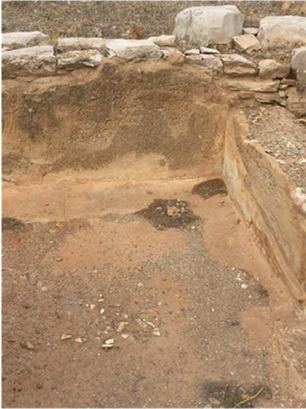
Fig. 1: Representative examples of the materials and the techniques used. Stone masonry and earth block masonry, both coated with thick hydraulic renders. The floors are made of various layers of hydraulic mortar. Stone masonry and earth block masonry constructed with earth mortars and plastered with hydraulic mortars constitute a building pattern (photo: N. Meimaroglou).
